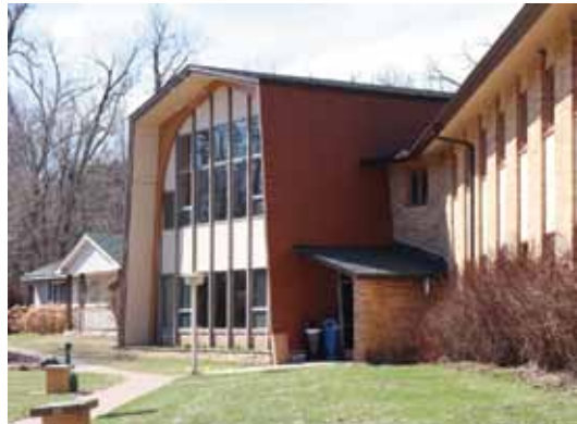
Completion of $64K mansard roof (destroyed in a 2017 hailstorm)
